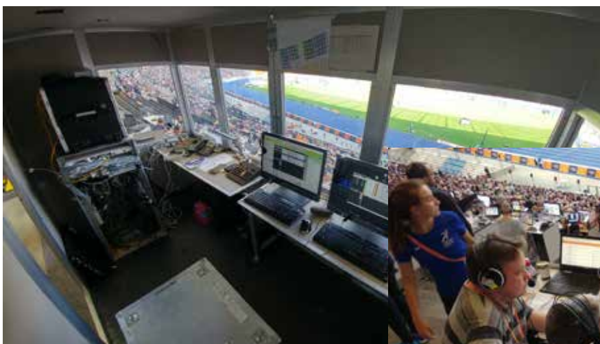
CCR with CCU (Commentary Control Unit) at the Olympic Stadium in Berlin during the 2018 European Championships.
